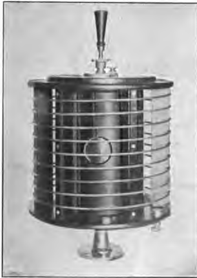
FIG. 6.—SPARK-GAP WITH MUFFLER, SURROUNDED BY INDUCTANCE.
